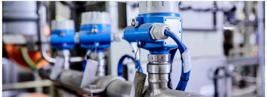
Liquiphant (compact vibration point level switch) used for leakage detection and to protect the hydrogen-cooled generator.
