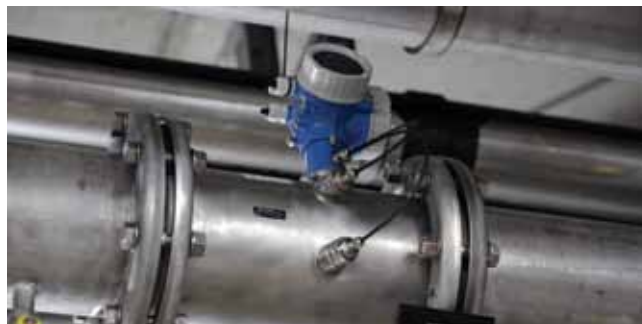
Ultrasonic measurement of biogas methane content and flow with the Prosonic Flow B 200
