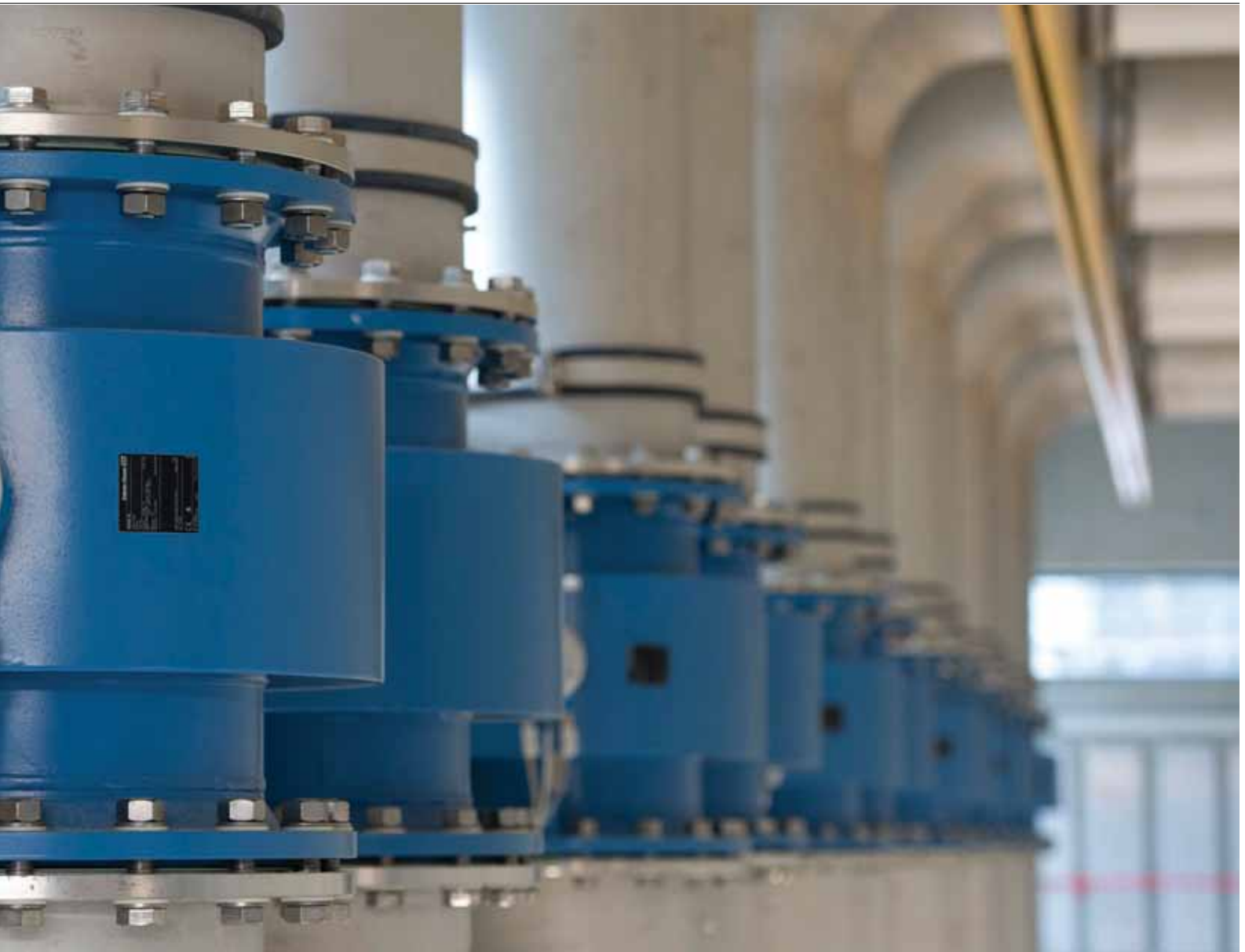
Flow measurement of water, wastewater or sludge: The electromagnetic induction method of flow measurement is the standard
