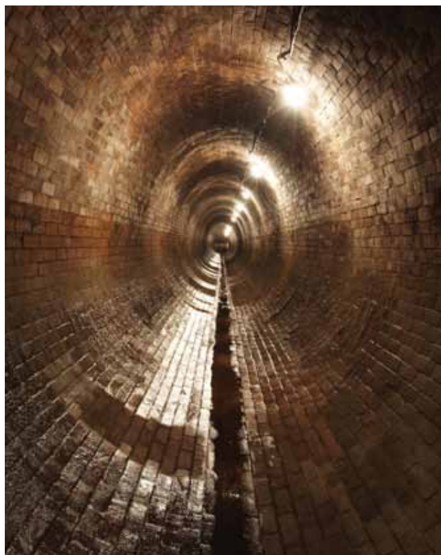
Inspection of a wastewater sewer for the safe channeling of water
